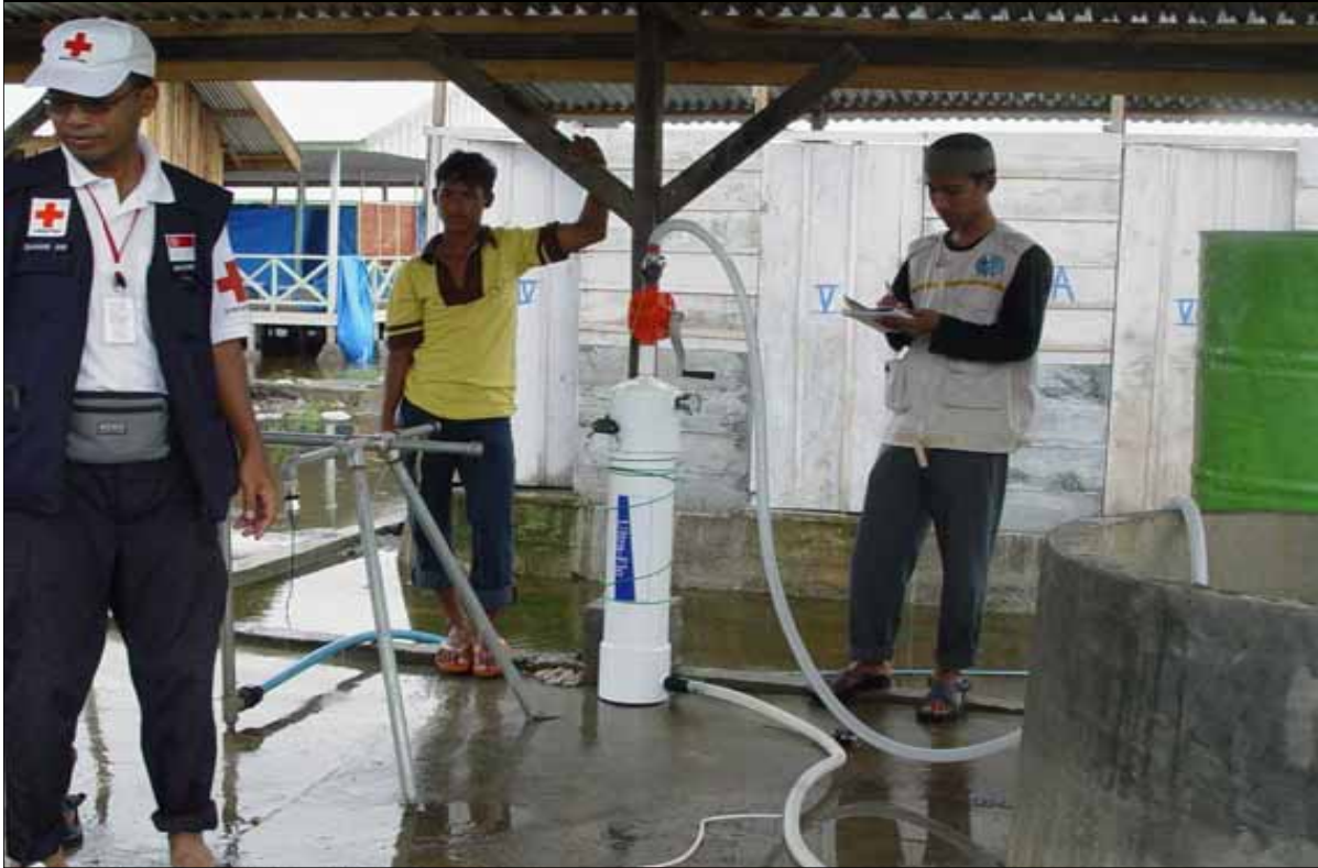
U660 WITH HAND PUMP BEING DEPLOYED BY RED CROSS IN REMOTE ACEH
