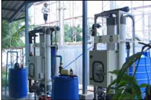
FIRST PILOT TESTING
