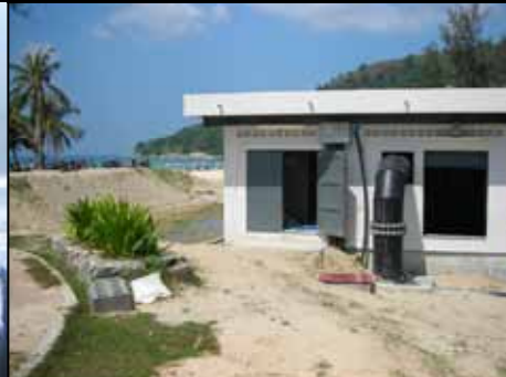
PUMPING SEAWATER UP THE MOUNTAIN TO SWRO PLANT
