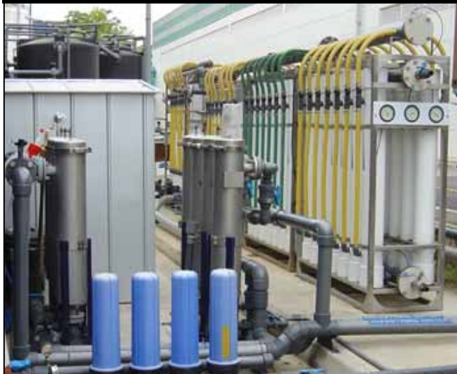
WASTERWATER UPGRADING & RECYCLING 2,000 m 3 /day
