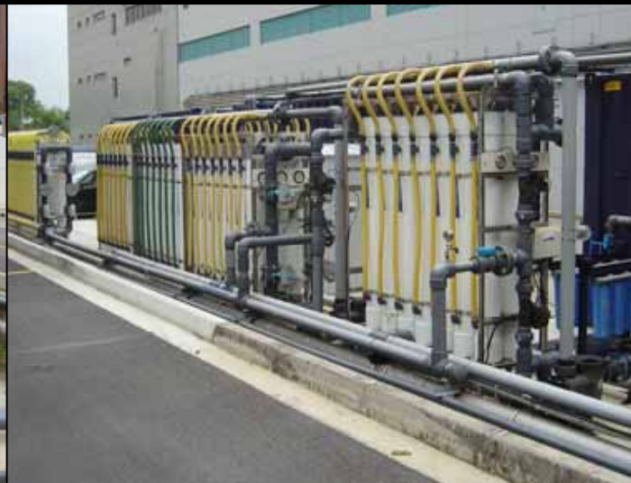
WASTEWATER 10X CONCENTRATION FOR INCINERATION 200 m 3 /day
