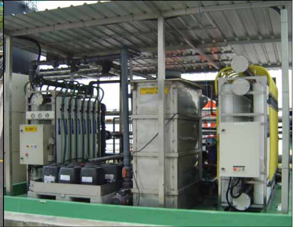
WASTEWATER 10X CONCENTRATION FOR INCINERATION 200 m 3 /day
