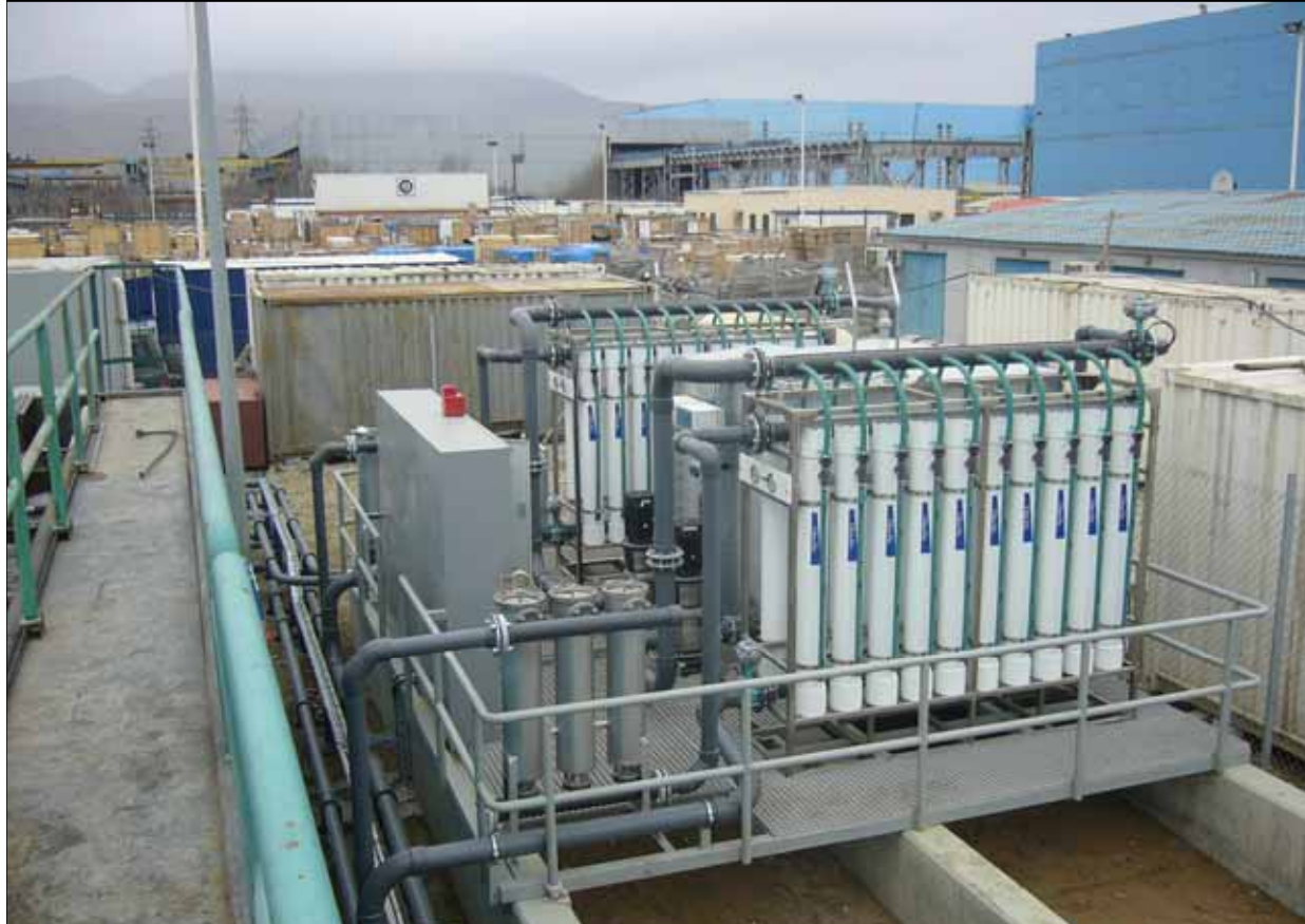
2 X M-20 SYSTEM PRODUCE WATER TREATMENT PLANT
