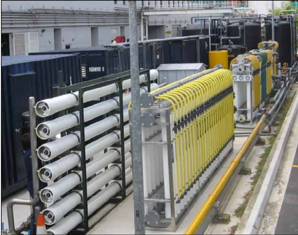
WASTERWATER UPGRADING & RECYCLING 2,000 m 3 /day
