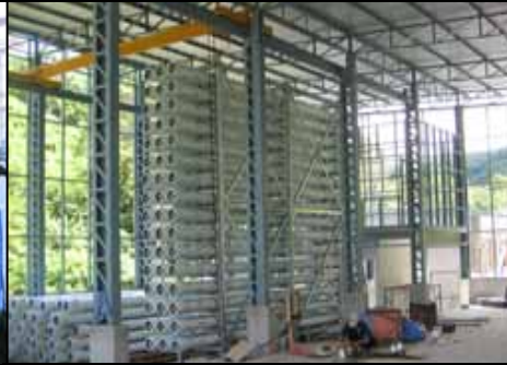
ASSEMBLING RO SYSTEM
