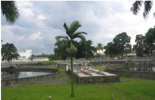
Stage 1 Incoming Industrial Waste from Clarifiers
