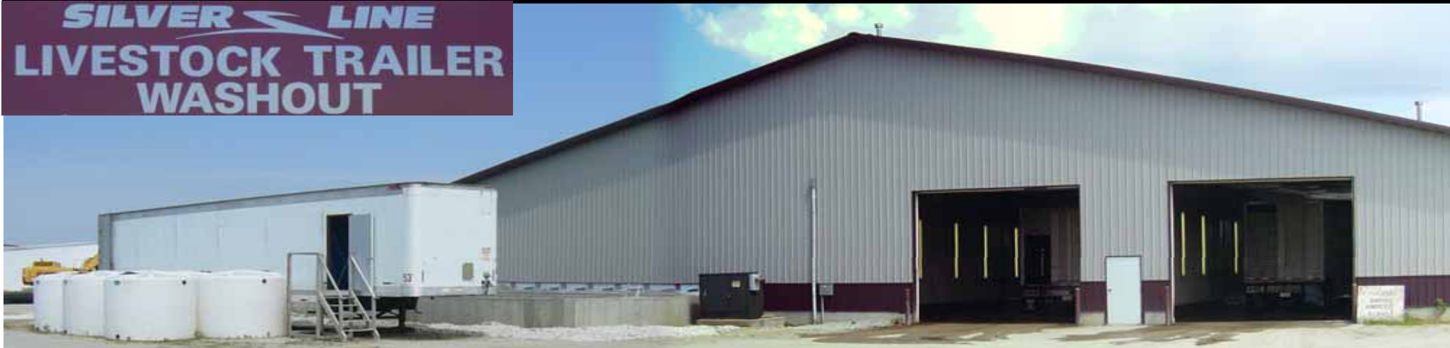
20ft container with MBR system for treatment of livestock washout wastewater in trailers to meet discharge standards and re-cycling for non-potable use
