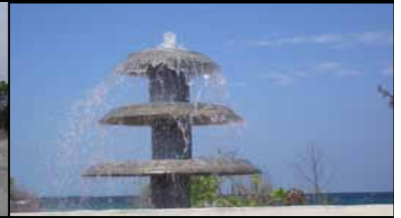
FEED WATER TANK FOR AERATION BEFORE MEMBRANE TREATMENT
